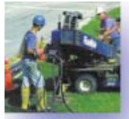
Figure 13: Underground trenching using FlowMole equipment. (Courtesy UtilX Corp, Kent, WA)
